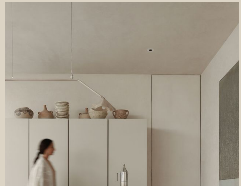
27. Roof finish Beige paste type pigmented stucco Brand: Kimiplaster (or similar) chukum color 3.07
