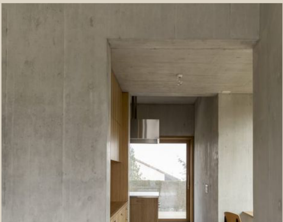
10. Wall finish Natural exposed concrete 1.01
