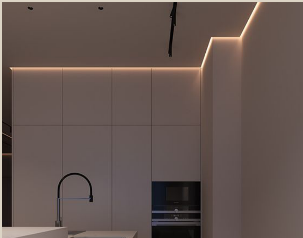
37. TL02 ALPIN LED luminaire power MAX 15W color aluminum 3000K warm light, integrated in detail of ceilings in apartment rooms
